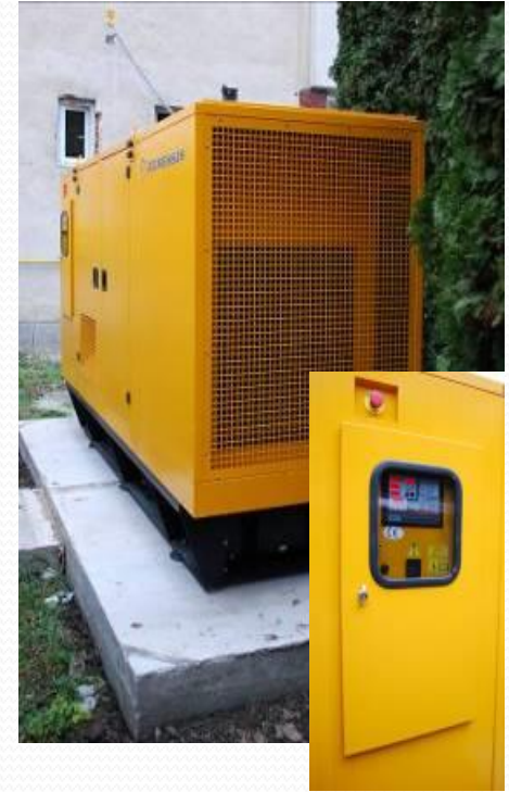
Power generator 275kW
